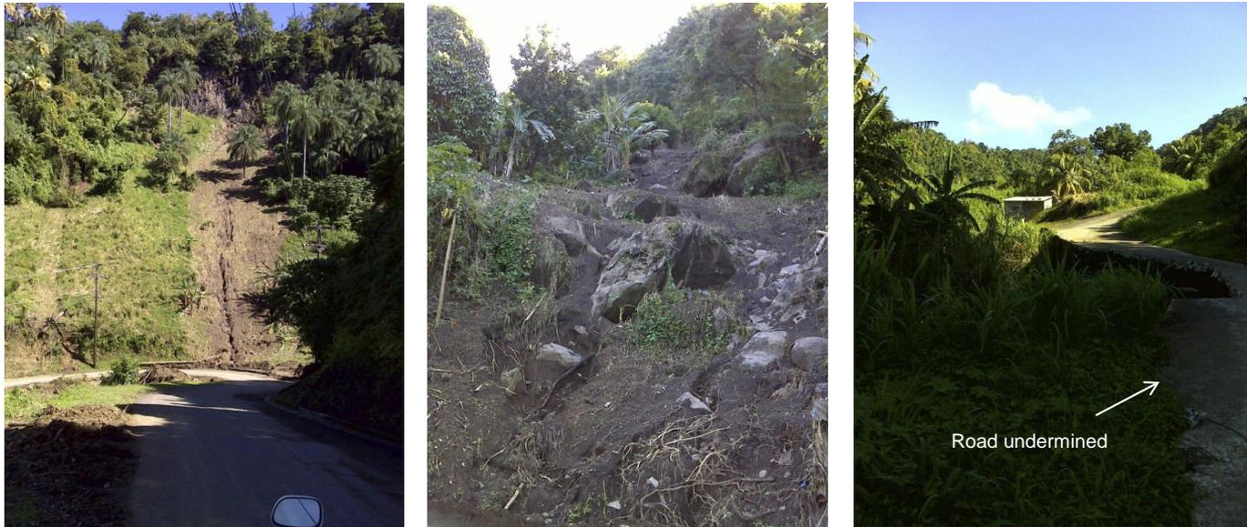
Figure 83: Evidence of landslides and land slippage along the Leeward Highway north of Dark View near N13.28751 W61.24955. Minor road at N13.29209 W61.23801 undermined and damaged.
