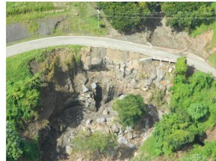
Partial failure of road support along the Windward Highway near Orange Hill caused by overland flow undermining the abutments.
